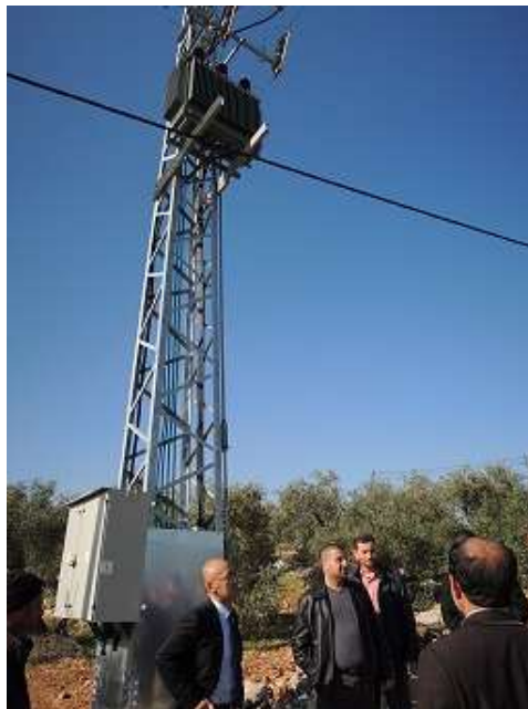
A new transformer installed to upgrade the electricity network at Seilat al Hariyeh
