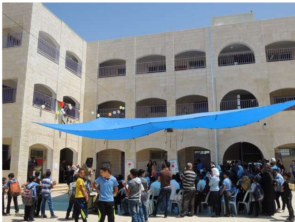
Second floor of Al Khass School constructed by the assistance of the Japanese Grant
