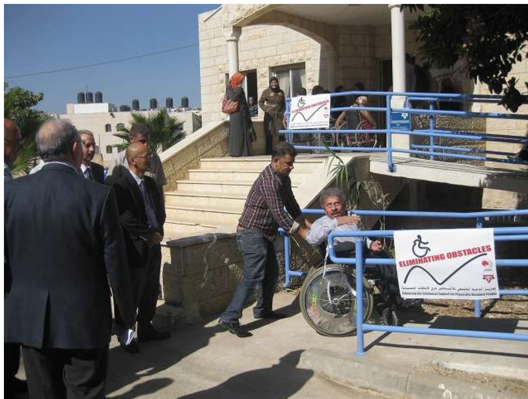
A handicapped man using the ramp and handrails newly built at the entrance of Bethlehem Sports & Youth Directorate
