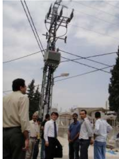
Rehabilitated Electric Network
