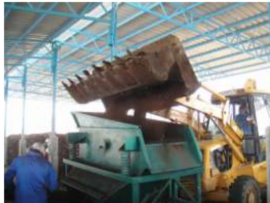
Constructed Compost Production Unit
