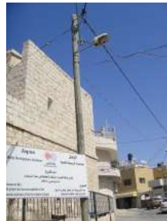
Newly Installed Electricity Network
