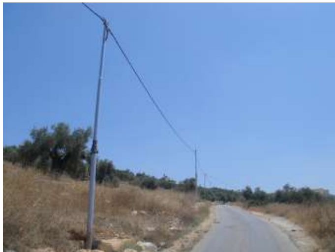
Newly installed electricity network
